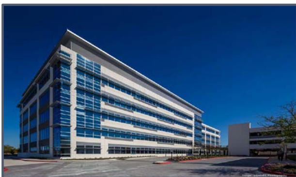
Offices at Greenhouse - Houston, TX KBS Growth & Income REIT November 14, 2016
